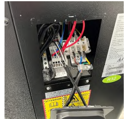
Fig.2 Electrical Panel Removal
