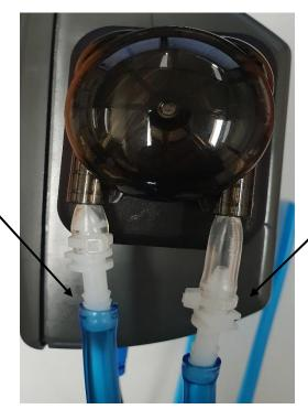
Injection Hose – goes from this side of the pump to the Injection Manifold.
